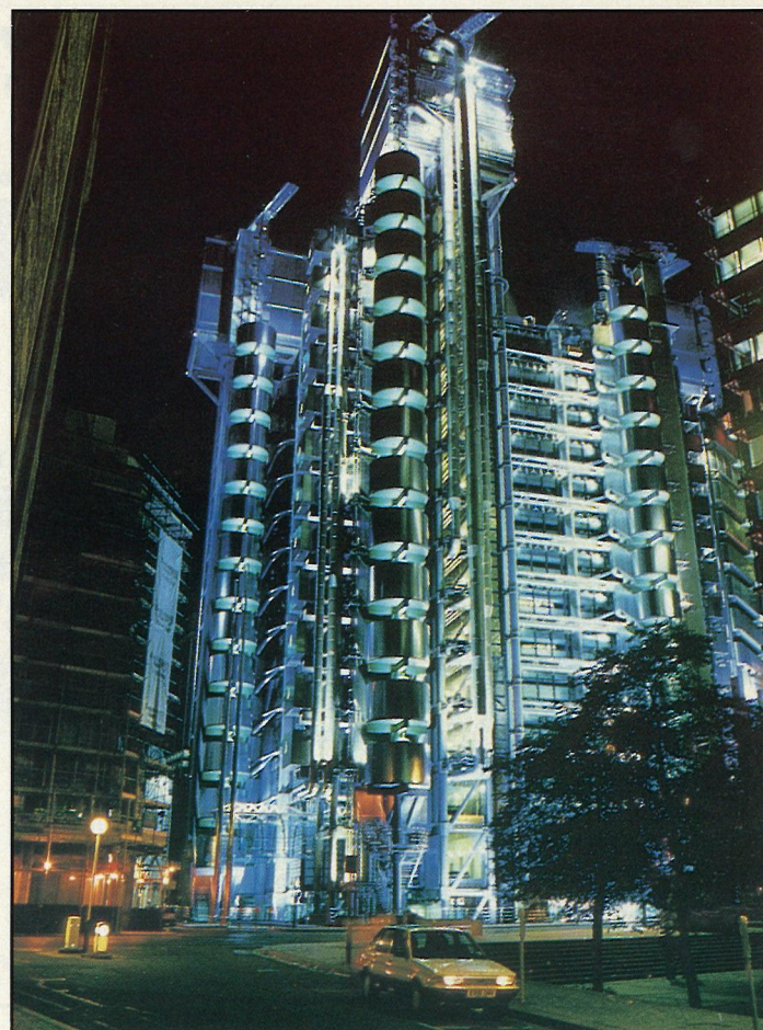
Specially doped metal halide lamps tint the metal cladding blue on the Lloyds of London building.
