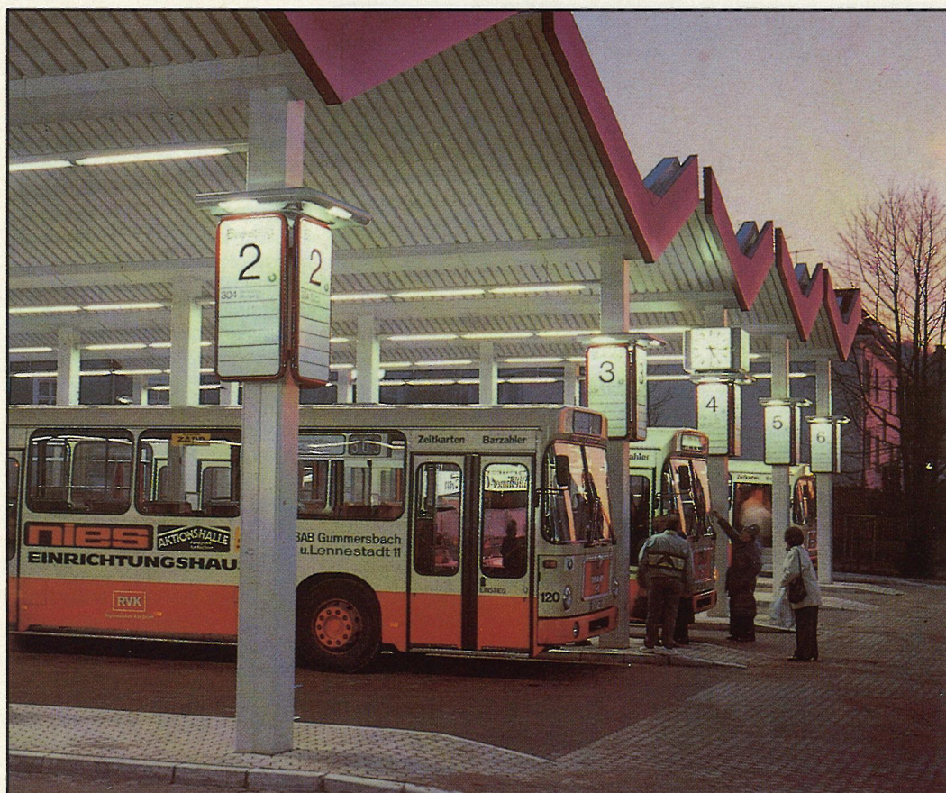
A modular linear lighting system used in a bus station.
